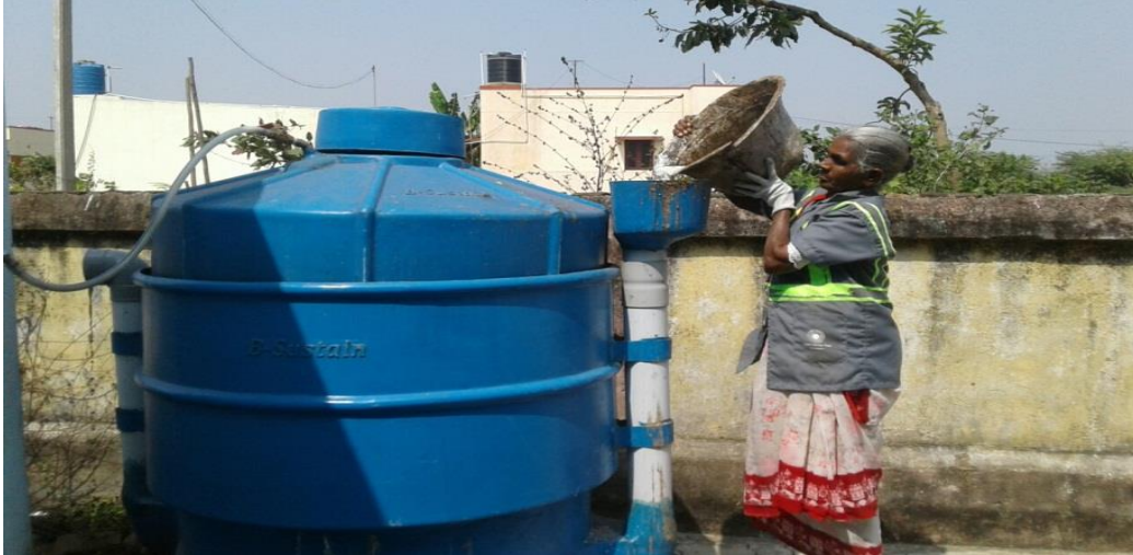
A Mini Bio-gas Plant in Shed where the waste is converted into gas
